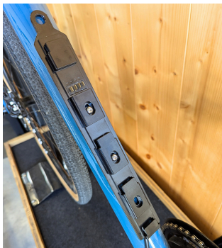
Installation conforme du rail
